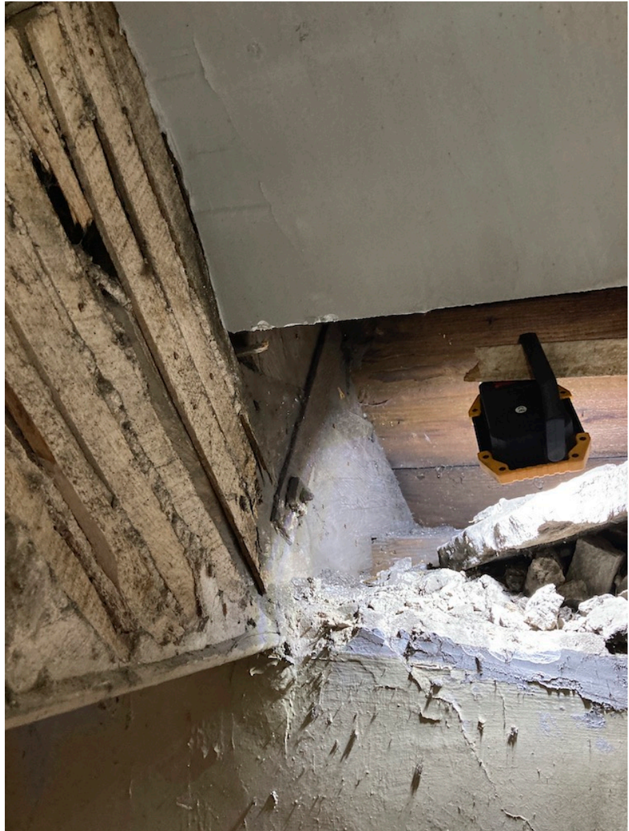
A typical truss bearing, this being the south end of the truss nearest the dividing wall above the main hall. In it you can see the lathing to accept a plaster coating and the edge bead of the timber applied to the underside of the beam. Also an iron bracket holding the rafter foot onto the beam. Note the plasterboard applied as part of a whole ceiling repair. © A. P. Rodger 2021
