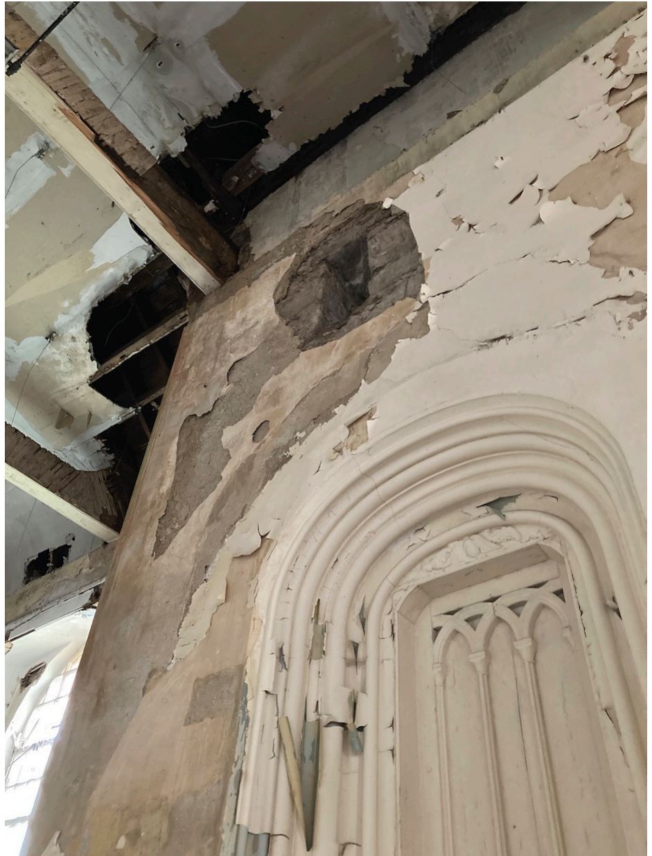
North wall of the tower in the main volume. It shows the recessed doorway from the tower into the now absent pulpit. It also shows the shot hole above but there is no obvious evidence of the timber canopy, as described by Macara. © A. P. Rodger 2021
