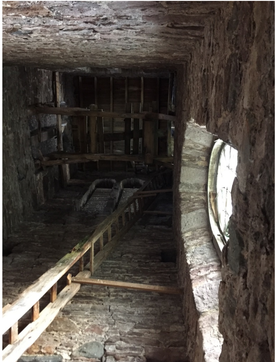
View of the tower from the mezzanine level © Andrew Rodger 2021. Note the running crack on the east wall which is replicated to a lesser degree on the west wall and which aligns, more or less, with the intersection with the main south wall outside face but also relates to the blind window cavities in the wall thickness.
