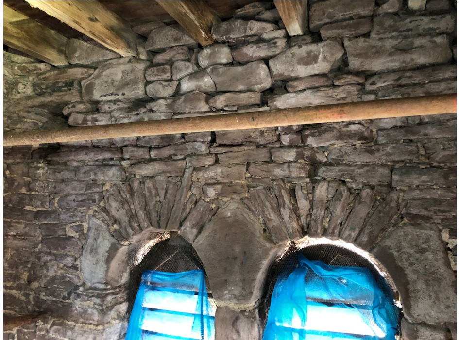
West wall of level 4 showing the unstable roof joist bearings © A. P. Rodger 2021
