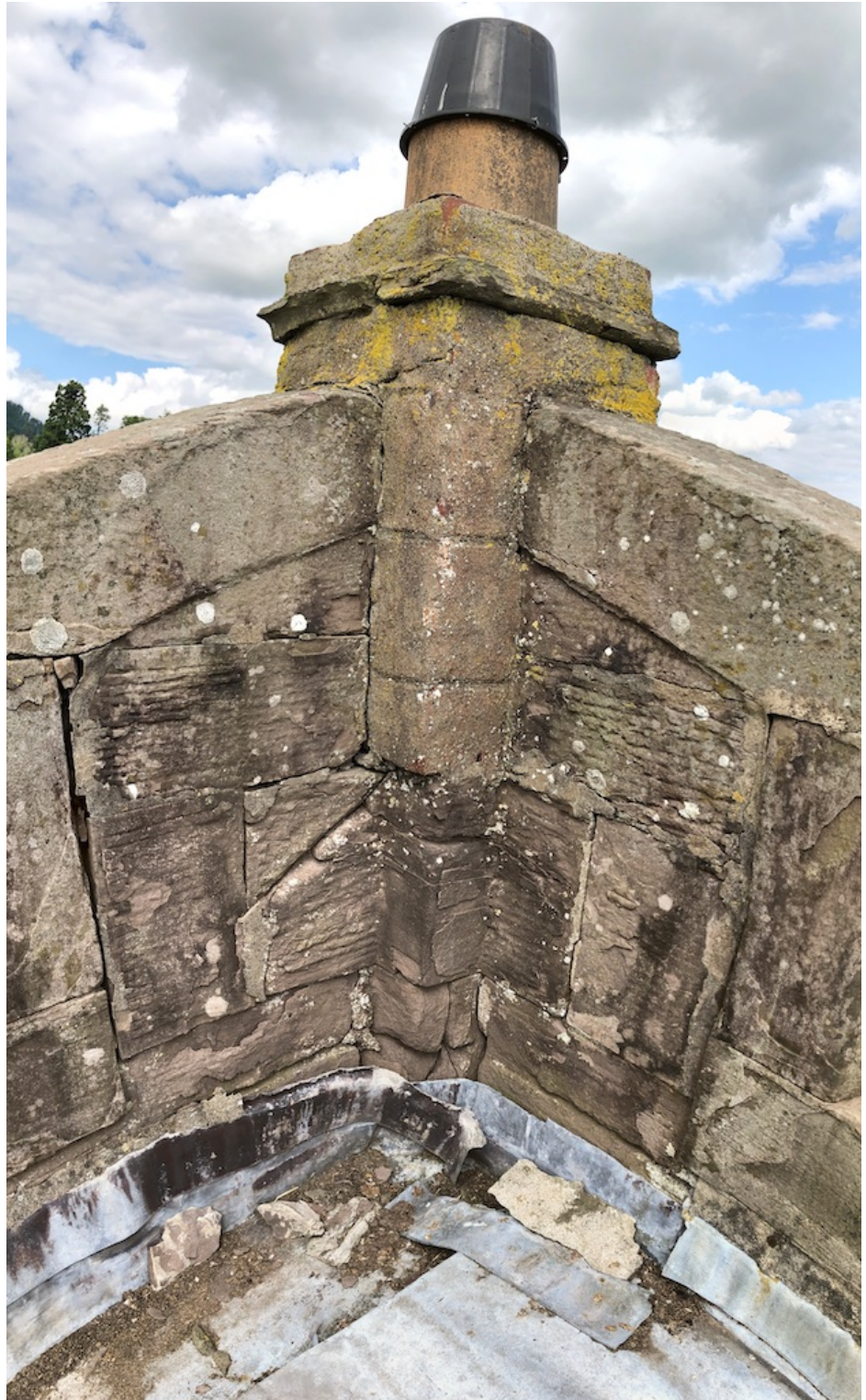
View of the north east corner of the parapet showing the rebuilt section. The only stone which bonding across the parapet is the broken one with its bed approx. 120mm above the raggle. Above this stone the pier is formed with unbonded brickwork. © A. P. Rodger 2021
