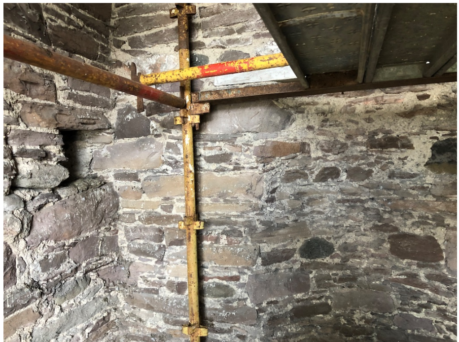
Level 3 view of north west corner of tower, showing typical putlog and the top of the curved recess in the north wall © A. P. Rodger 2021
